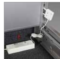
Step Four: Plug Power Terminal into gondola and driver into outlet
